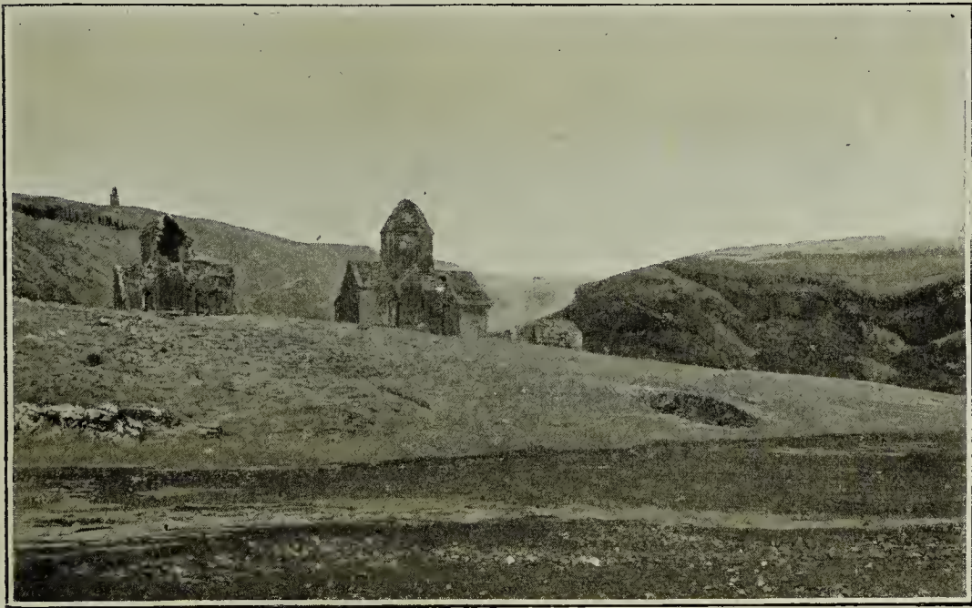
FIG. 94. KHOSHA VANK: CHAPELS IN THE RAVINE OF THE ARPA CHAI.
